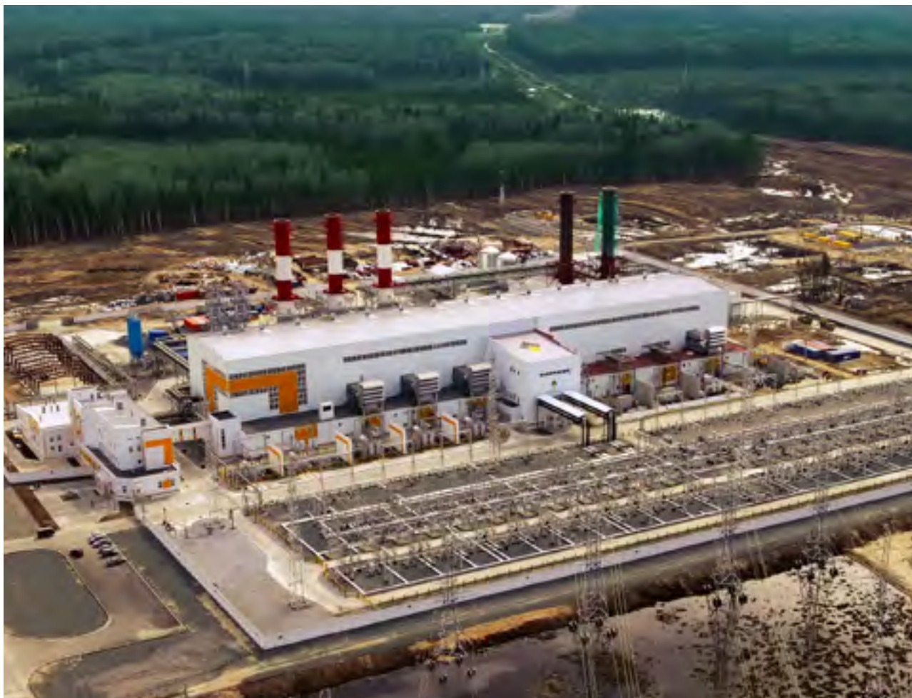
D Western Siberia, KhMAD. Gas-turbine power station at the Priobskoye field
