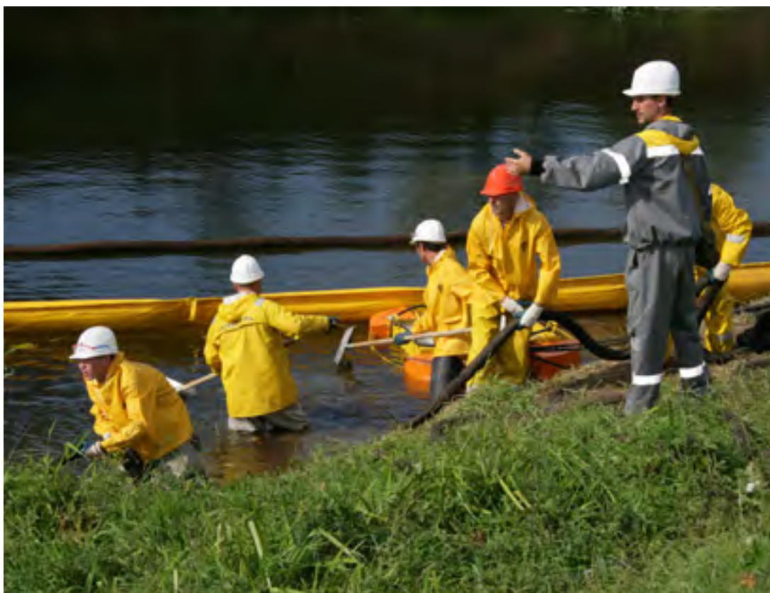
Republic of Udmurtia. Emergency response exercises at Udmurtneft
