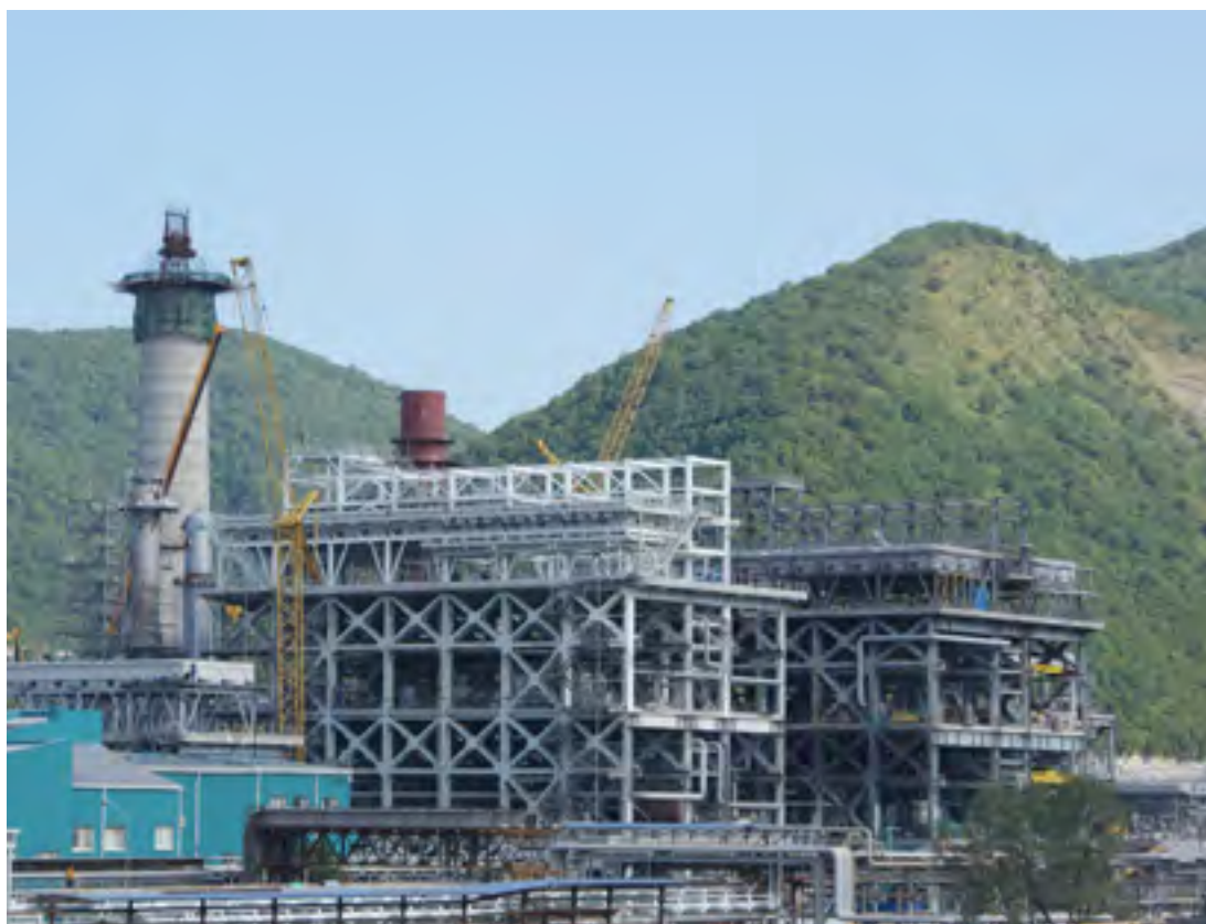
D Tuapse Refinery. Construction of an atmospheric and vacuum distillation unit
