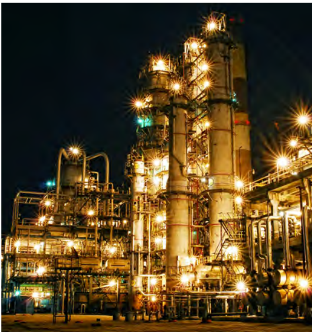
D Syzran Refinery. Atmospheric and vacuum distillation unit
